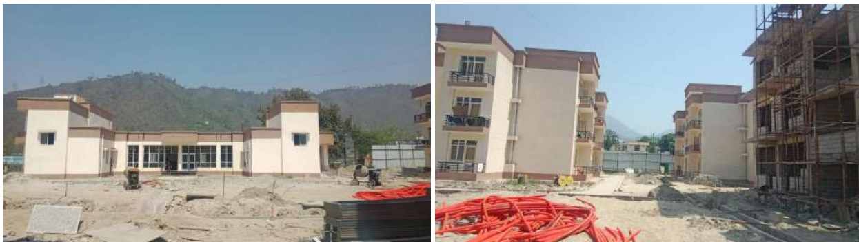
Construction Activities of Phase – I
